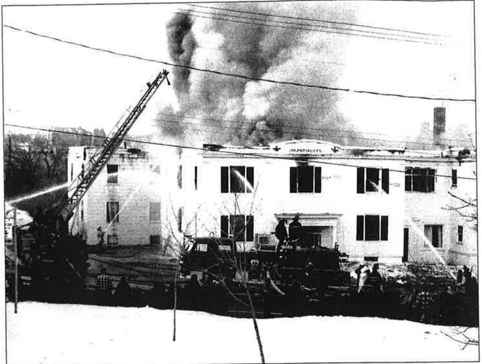
Fire breaks out at the Oak Hotel.
